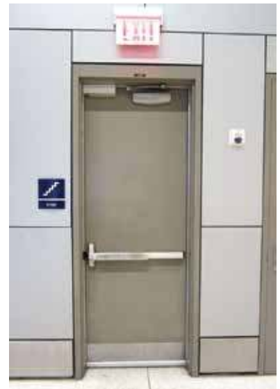
Mag-locks released by hardware mounted on the door are addressed in a separate code section from mag-locks released by a sensor.
