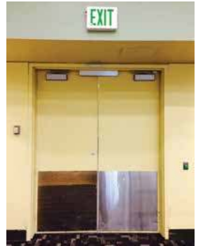
The section called Access Controlled Egress Doors has been changed to Sensor Release of Electrically Locked Egress Doors in the 2015 IBC.
