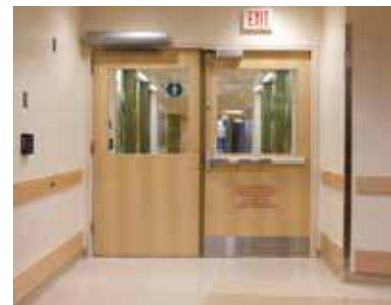
In the 2015 edition of the IBC, the activation time for delayed egress locks has changed from 1 second to 3 seconds, which is consistent with NFPA 101.
