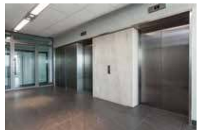
Electrified locking of elevator lobby doors is only addressed by NFPA 101, not the IBC, although some jurisdictions have adopted code modifications that allow it.
